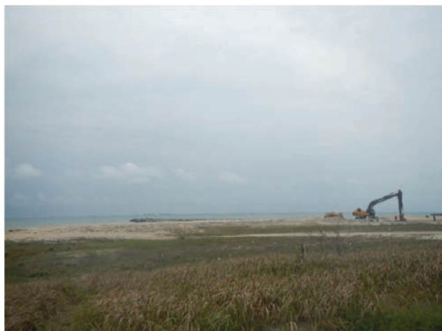
Figure 5. Construction activities at Elegushi Beach in September 2013.
